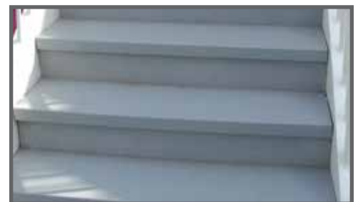
Covered stair treads, with hidden hold down clips, lead to a water slide at a municipal waterpark in Oklahoma.
